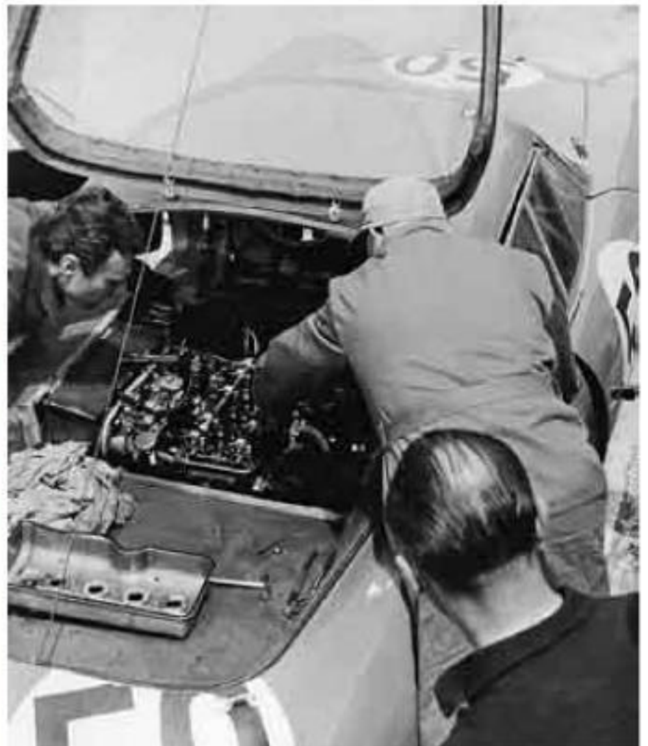
The double overhead cam Gordini engine. (Photo GB)
